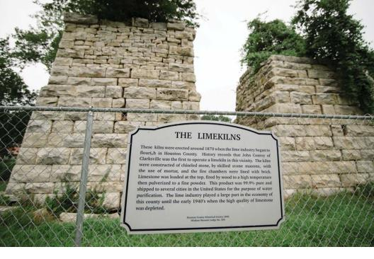
Water purification for Houston in the late 1800s began with limestone pulverized in the lime kilns. Constructed of chiseled stone by skilled stone masons around 1870, fire chambers lined with brick allowed the high temperatures necessary to create a fine powder, 99.9 percent pure. Several cities in the United States of America used the lime through the 1940s when the high quality of limestone in the area was depleted.
